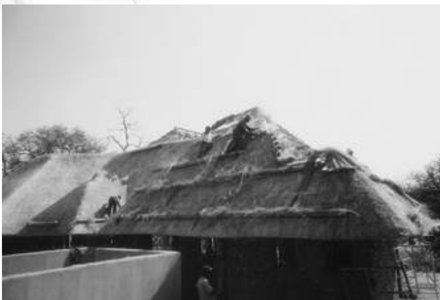
Photograph 6 Completing the thatching at the ridge of the roof
