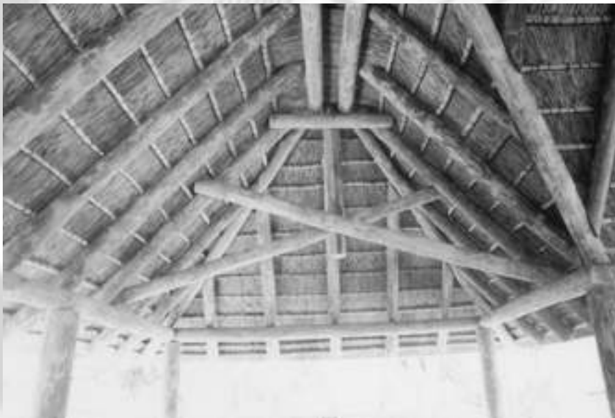
Photograph 11 Typical scissor-type truss configuration
