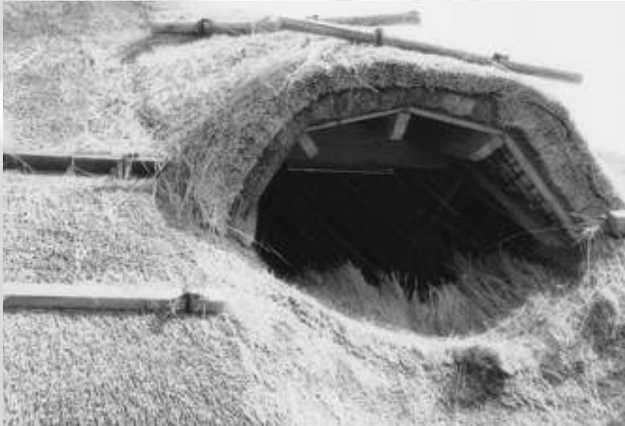
Photograph 10 Typical thatched-roof dormer window under construction
