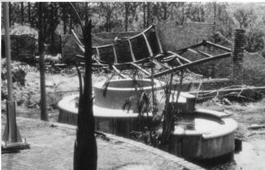
Photograph 17 Severe warping of structural steel, an indication of extreme heat
