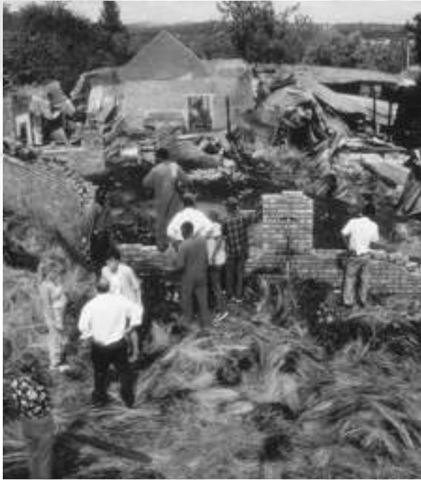
Photograph 16 Total destruction, following a thatch roof fire
