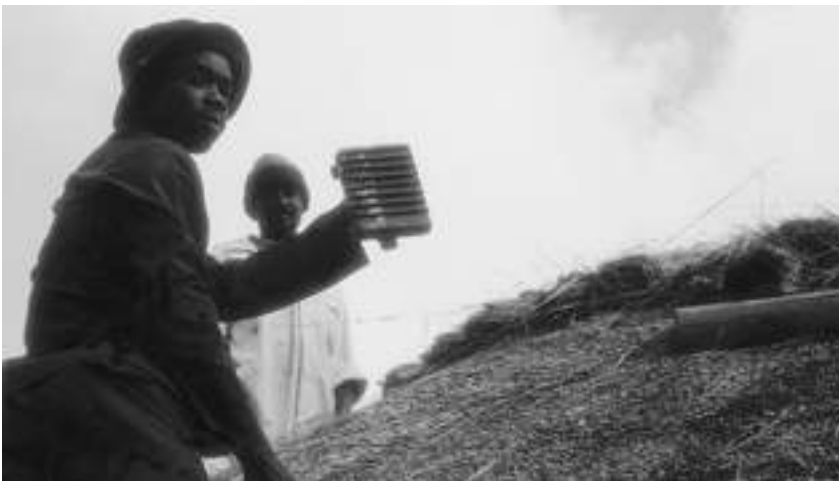
Photograph 3 Thatching spade or leggatt ("dekspan")
