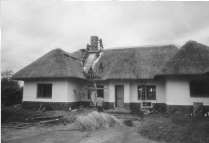
Photograph 7 Chimney (with flashings) at ridge of roof
