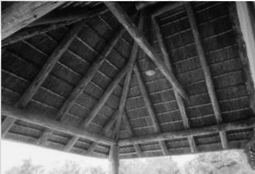
Photograph 13 Typical thatched-roof hip detail
