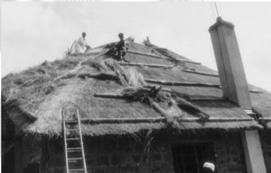
Photograph 5 Typical two-man thatching team with helper (one team member on the inside)
